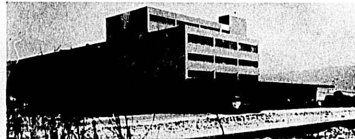
New Migros macaroni manufacturing plant at Buchs.
